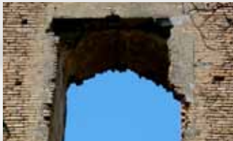
Šarengrad, 15. st. – ulazna kula, ostaci pročeljne žbuke oko prozora Šarengrad, 15th century – gatehouse, remains of plaster around the window
