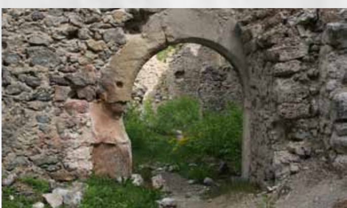
Ružica grad, kraj 15. st. – portal s polukružnim nadvojem Ružica town, late 15th century – portal with semicircular lintel
